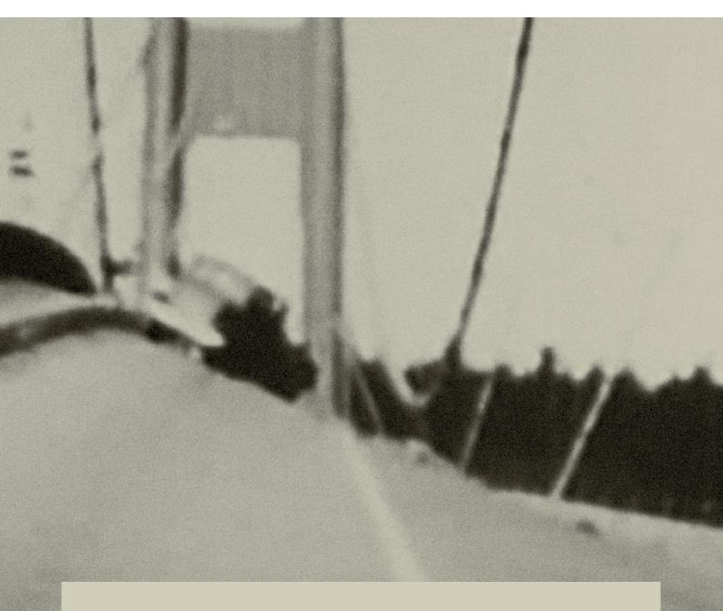
Resonances occur when a system capable of vibrating is set into vibration by an external influence, the frequency of which matches the system's own. The vibrations intensify, and – for instance – harmonious sounds can arise.
